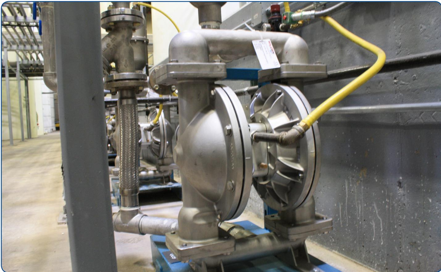
Advanced Air Distribution System (ADS) technology can reduce the operating costs for air-operated double-diaphragm (AODD) pumps in a number of industries, including chemical processing, food and beverage, oil and gas, pharmaceuticals and mining.
