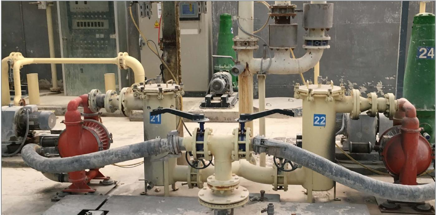
The constant motion that the diaphragms in an air-operated double-diaphragm (AODD) pump are in during a fluid-transfer operation puts them at risk of degradation and breakdown. However, a new integral piston diaphragm (IPD) design protects the diaphragm from failure while still delivering expected flow rates, efficiency, consistency, abrasion resistance and operational safety.
